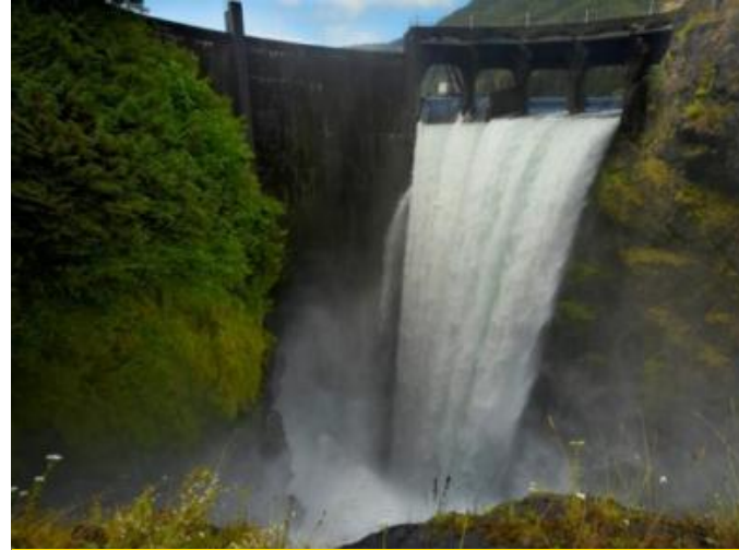
Glines dam before removal Elwha River © John Gussman, Return of the River / Patagonia
