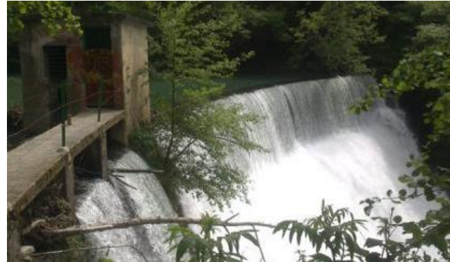
Inturia dam before removal © Basque Water Agency)
