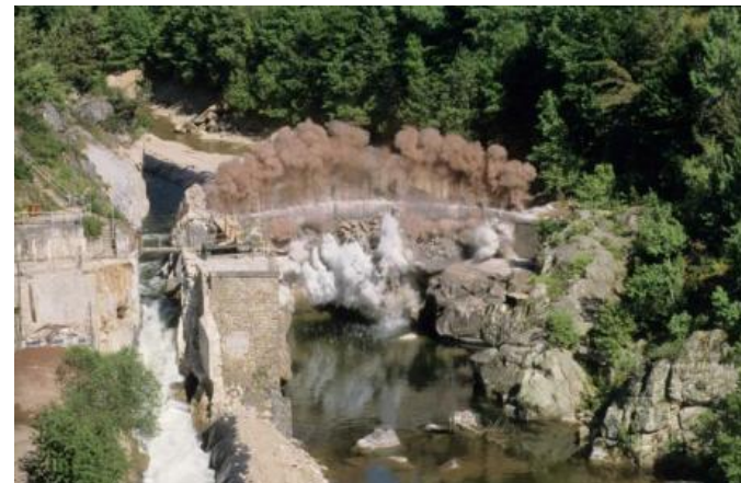
Saint-Etienne-du-Vigan dam removal works © ERN, Roberto Epple
