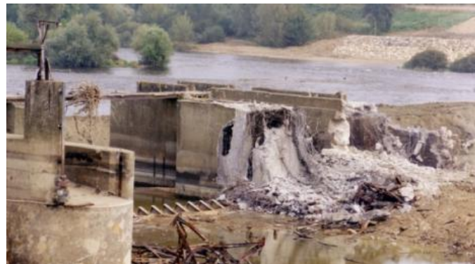
Maisons-Rouges dam removal works © ERN, Roberto Epple
