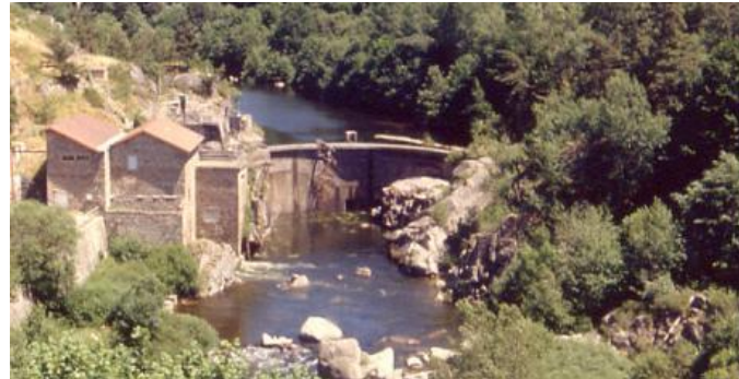
Saint-Etienne-du-Vigan dam before removal © ERN, Roberto Epple
